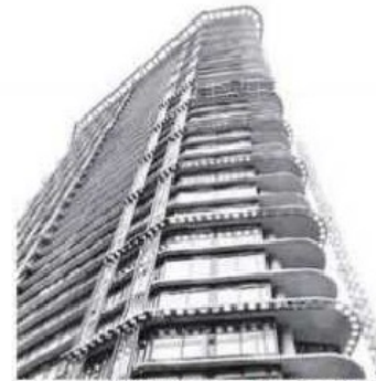
Ornamental ironwork on the facade of the W Tower is intended to handle ivy that will provide cooling for the structure. Photograph by: Ian Lindsay, Vancouver Sun
