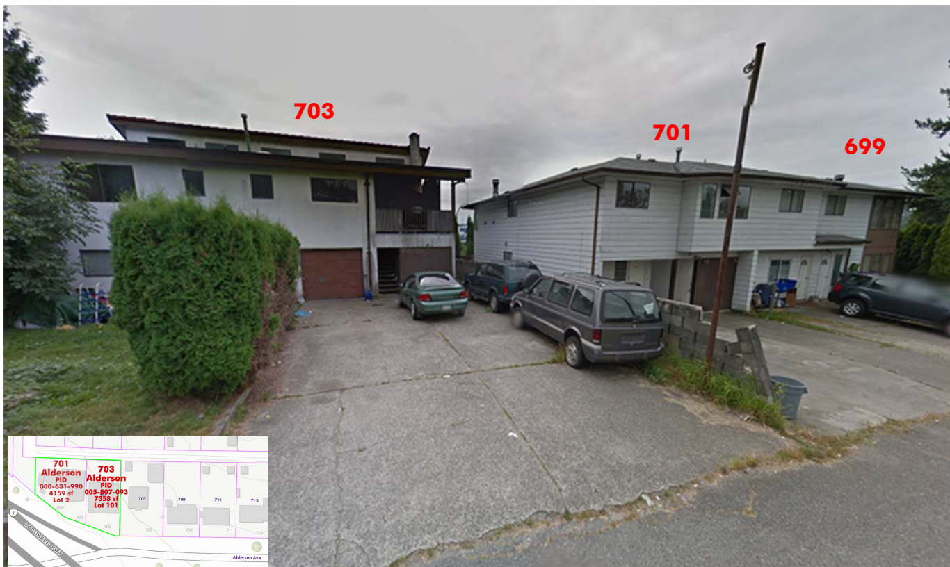
Alderson Avenue Homes
