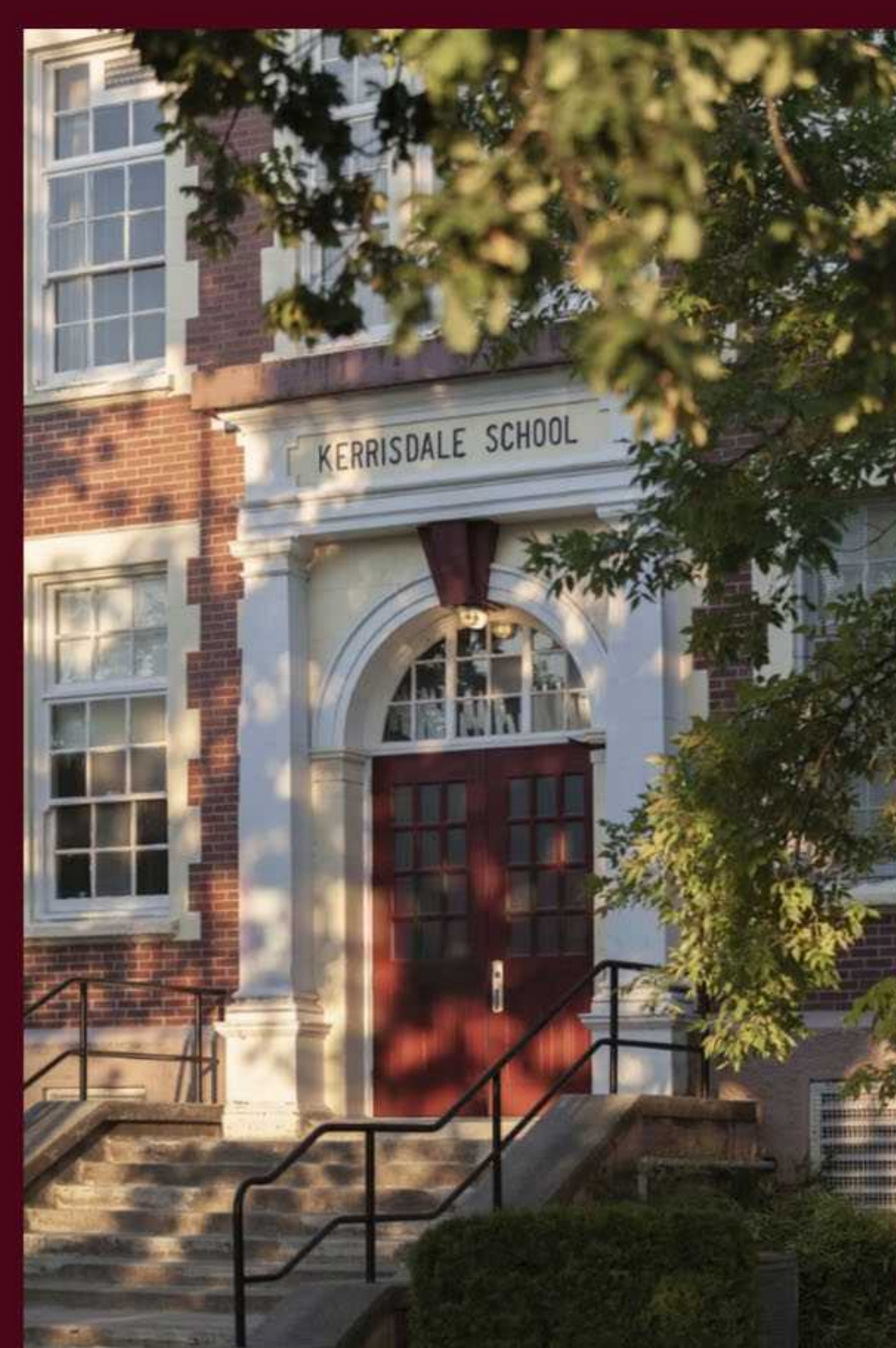
KERRISDALE ELEMENTARY SCHOOL
