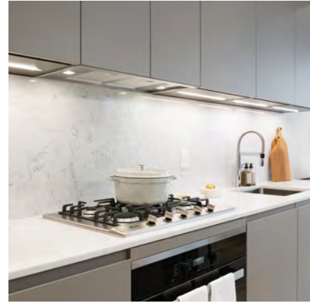
Continuous solid-slab backsplash
