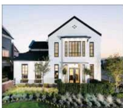
The owner-shared Dominion House is part of the project; it includes a children's play area, media centre, fitness rooms and entertainment space with a kitchen.
