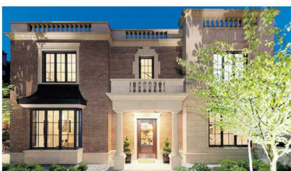
Residences feature concrete construction with brick cladding, columns and sandstone trim and balustrades. Photograph by: Wayne Leidenfrost, PNG Files, Special To The Sun
