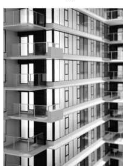
The alternating, offset balconies provide open and shaded areas for each unit.
