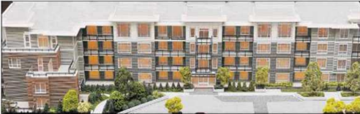
The exteriors at Elements, will be fitted with brick and HardieBoard siding and finished in an earth-tone palette.
