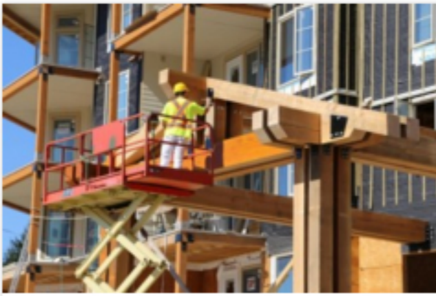
8 Photos Englewood Building Progress Sept 15
