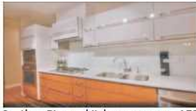
In the Ginger kitchens are an AEG cooktop and convection wall oven; an LG 24-inch refrigerator with bottom freezer; a Fisher & Paykel dishwasher; a Panasonic microwave; and a Broan slide-out hood fan. Slabs of quartz top counters and glass backsplashes face the walls between counters and upper cabinets. Bamboo flooring is underfoot in the kitchen, living and dining spaces and the master bedroom.
