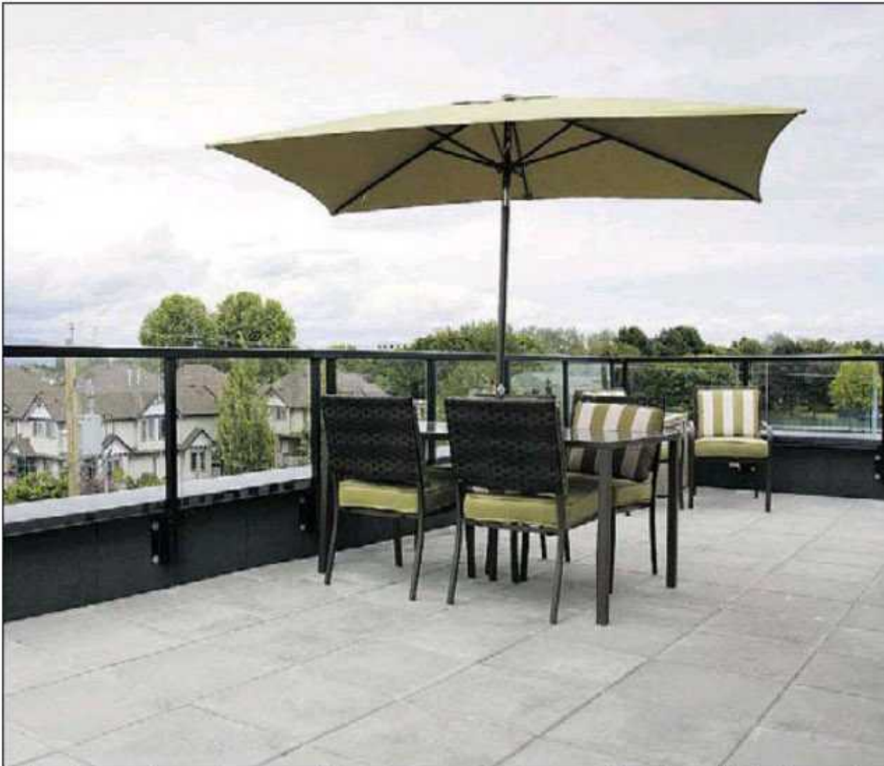
Rooftop patios at Steveston Views have gas hookups, and cedars will define each home's space. Corner-unit patios are a spacious 500 square feet, reports the project's Tussy Berg.
