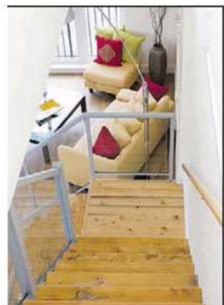
Reclaimed timbers and glass/metal railings were used for the Steveston Views' staircases. The homes have open floorplans and windows that rise to between seven and eight feet.
