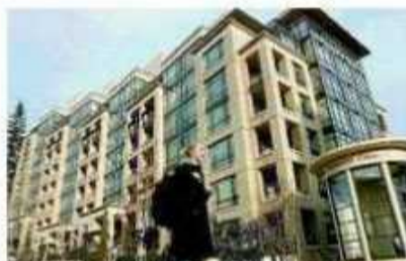
CREDIT: Mark van Manen, Vancouver Sun Definitely not a college dorm, the lower of the two One University Crescent buildings ascends Burnaby Mountain and asks the question, does the higher of the two descend the mountain? The expansive glazing makes the most of the views and permits the circulation of natural light and breezes into the apartments. A two-storey lounge (bottom right) anchors the southwest corner of this building, signalling the location of the One University Crescent common facilities, a private health club, billiards room and library. A gatehouse is located between the two buildings, at the entrance to the underground parking.
