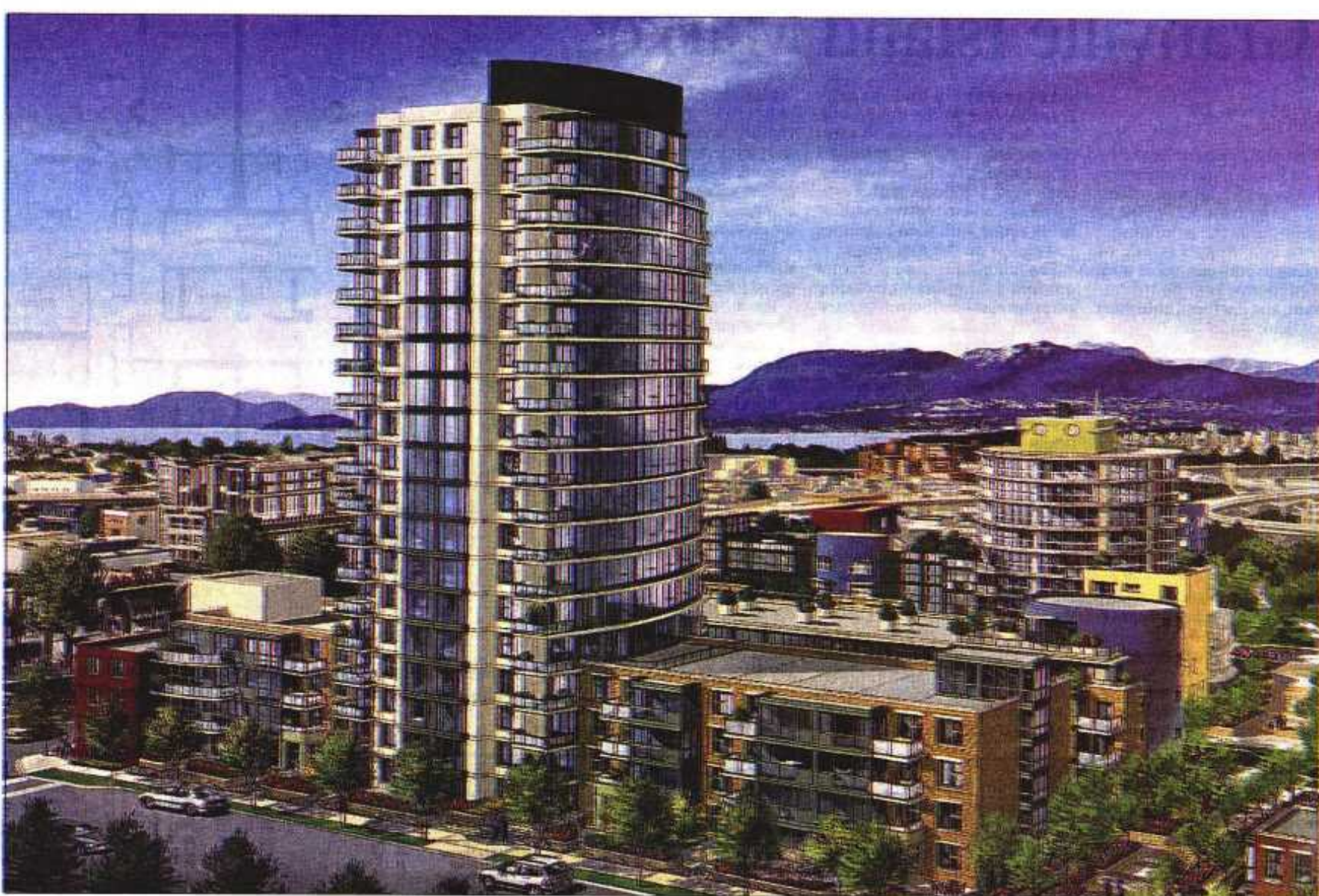
The Verona occupies the old site of Pacific Press, strategically close to Granville Island Market and the Broadway Corridor.
