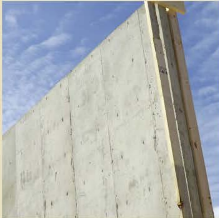
Industry-leading construction innovations including soundproof concrete common walls with an STC rating of 70 that set new standards
