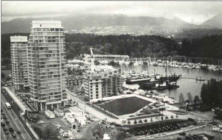
CONSTRUCTION CONTINUES ON THE WATERFRONT RESIDENCES AT BAYSHORE.
